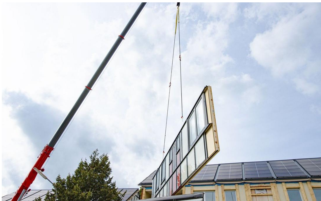
Figure: Example of off-site projects
