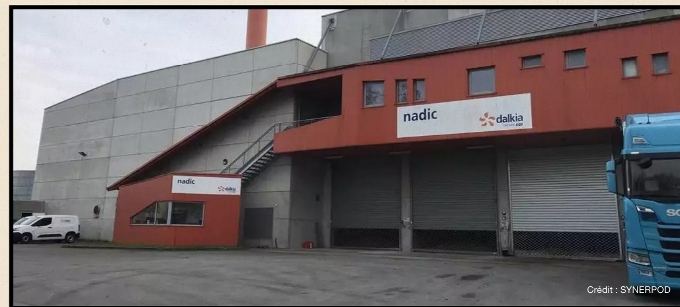
▲ Biomass boiler room, operated by Cléa, a subsidiary of Dalkia, which supplies the Bellevue-Chantenay network
